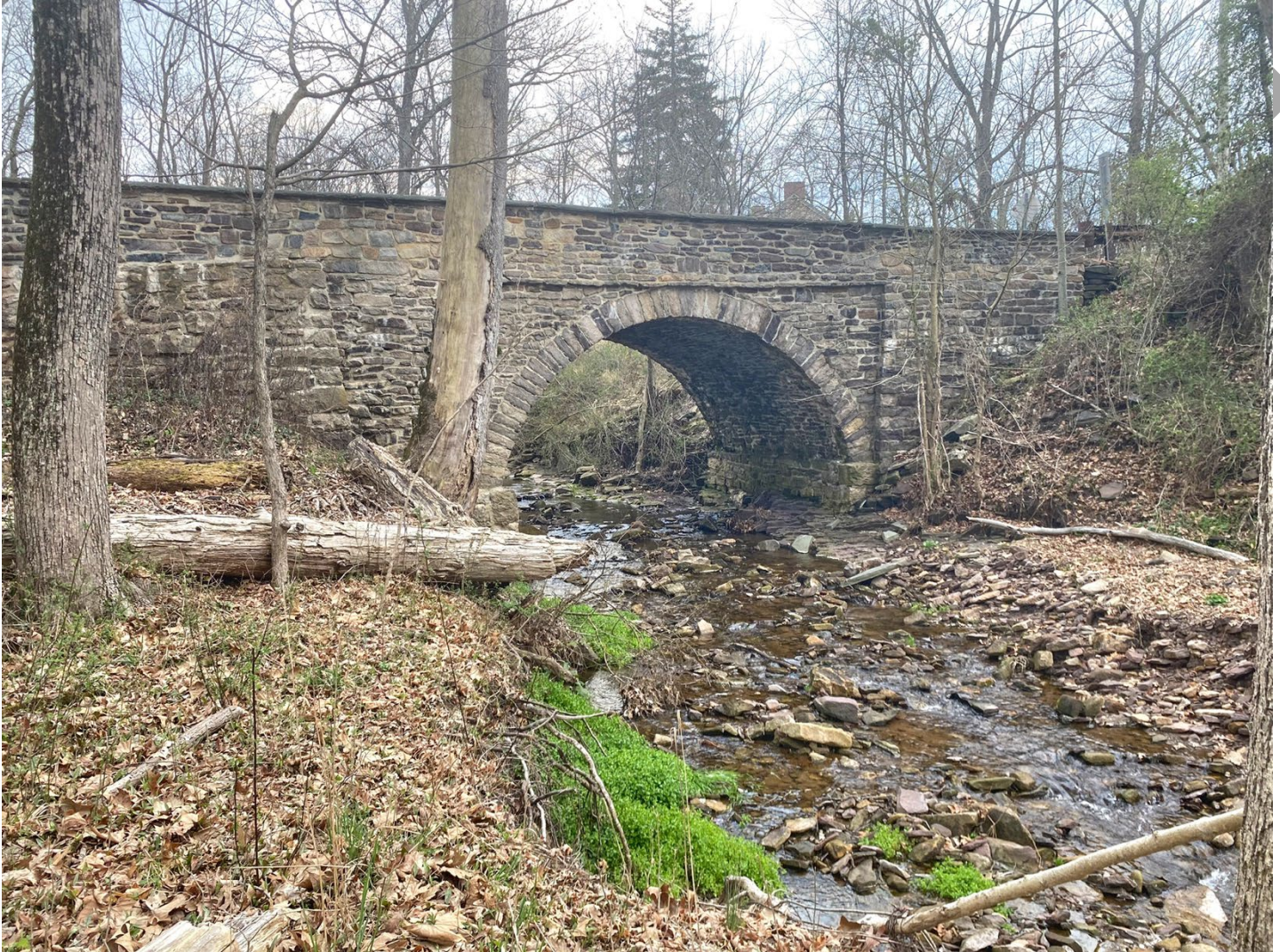
Photo 7: West (downstream) side of the Cold Water Bridge, View facing southeast.
