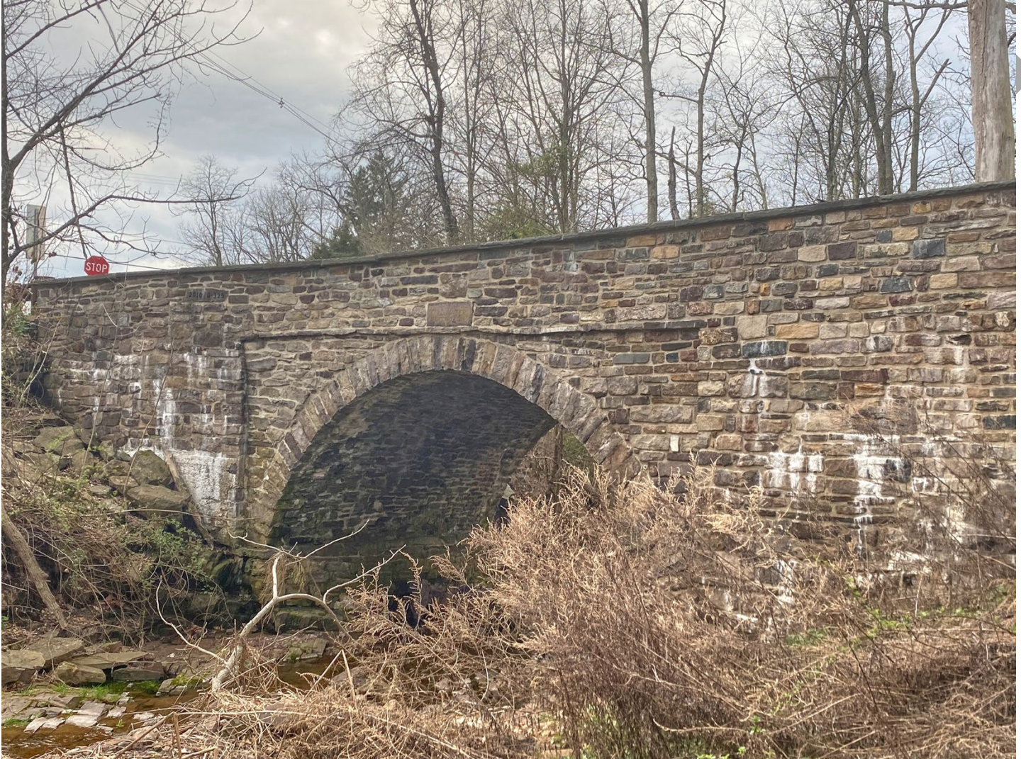
Photo 3: East (upstream) side of the Cold Water Bridge, View facing northwest.
