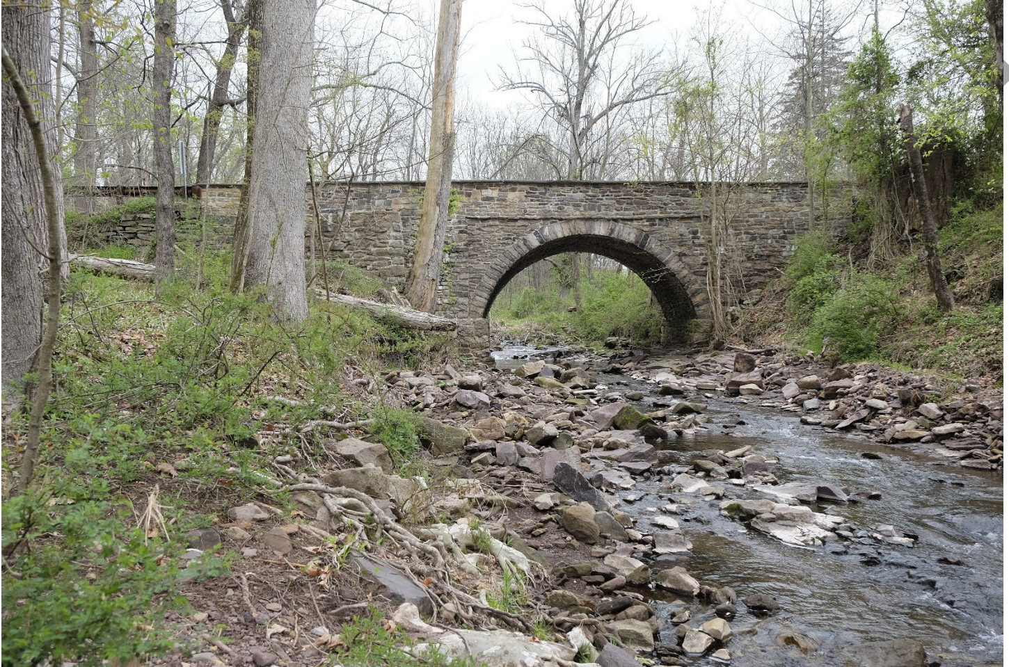
Photo 6: West (downstream) side of the Cold Water Bridge, View facing east.
